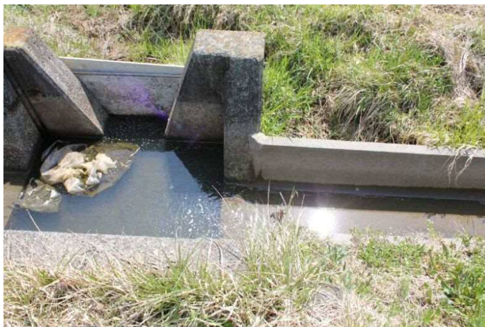
Fig. 2-2 排水路柵の外観 Outlines of pit in drainage canal
